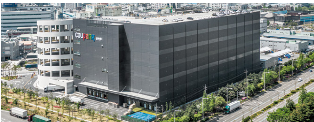
Bucheon Cold Logistics Park
