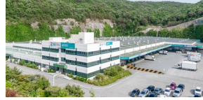
Gimhae Logistics Park 1 GFA 25,733m 2 | Completion 2000.12
