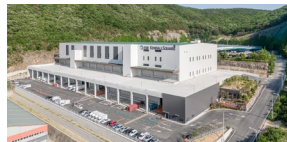
Gimhae Logistics Park 2 GFA 39,941m 2 | Completion 2019.12
